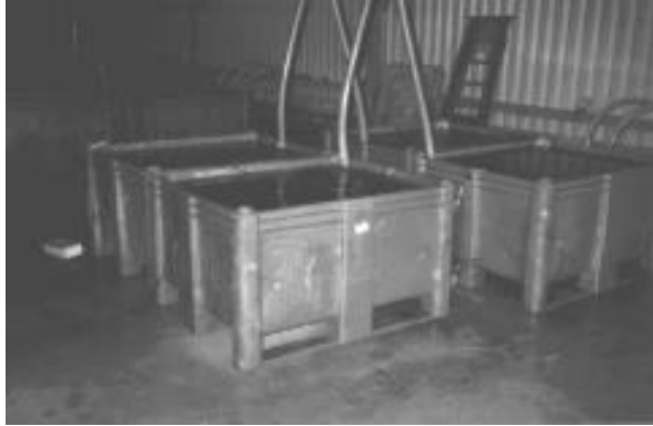
Bin and feed pipes in position
