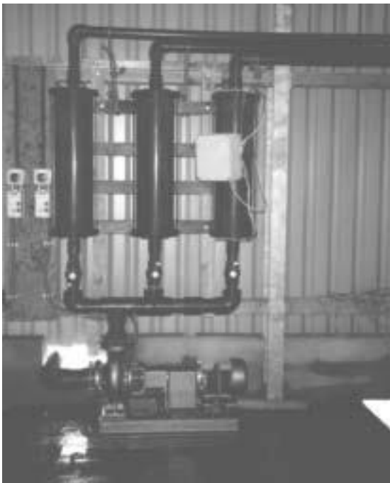
Pump and 3 x 6 lamp UV sterilisers
