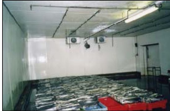
Figure 5 - An example of a simple spray water system for thawing fish blocks
