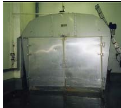
A forced air thawing unit in operation
