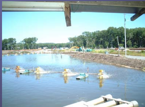
Floating aerators to provide oxygen
