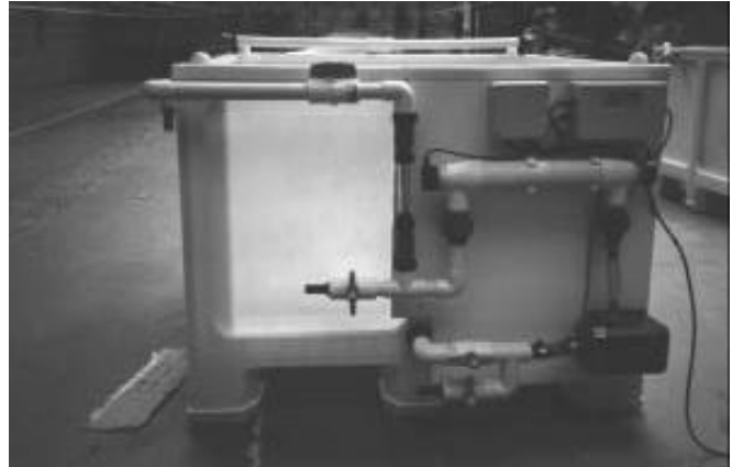
Panel mounted seawater recirculation equipment
